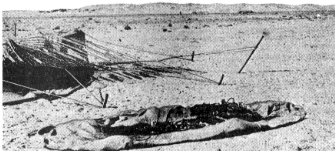
Figure 74. Another method to simulate an entrenchment is to place burlap or cloth in the outline desired and then fill in the simulated excavated portion with waste oil, paint, or scrapes of dark material. Note that the simulated parapet is formed by rolling under the edges of a large piece of burlap and creating the illusion of the mound of a parapet by piling sand under the burlap edges. The excavated portion of the slit trench is simulated in this figure by waste oil and dark colored salvage scraps.
